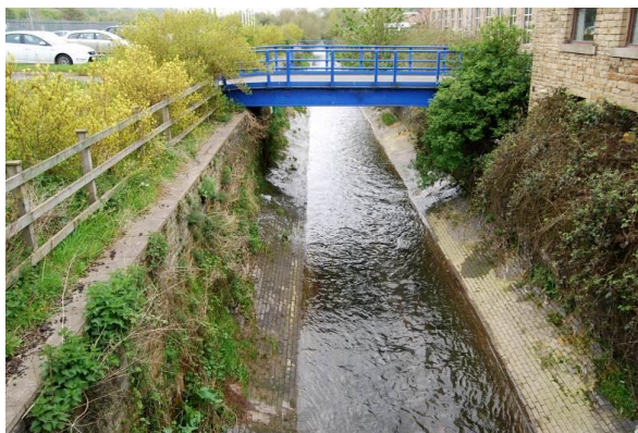
Figure 6. the Poplar Road bridge, looking upstream.
